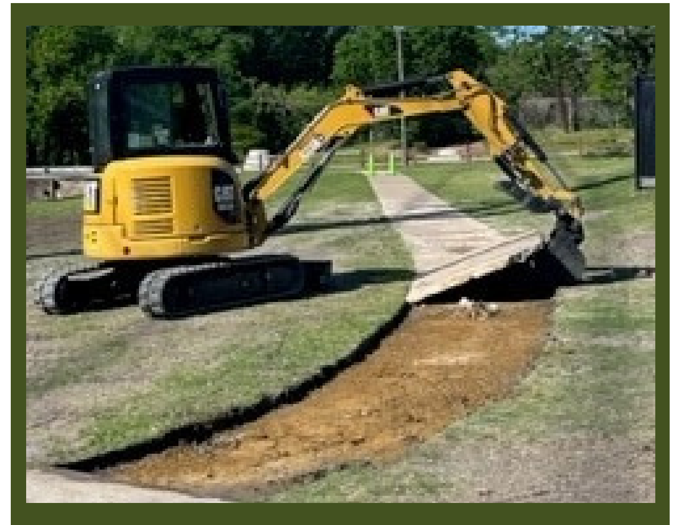
HARRY MYERS SIDEWALK REPLACEMENT
